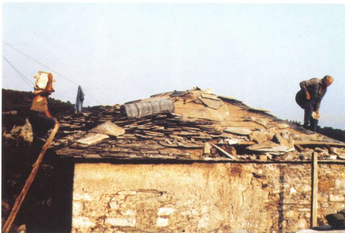
Master Stavros Kornoutos with an apprentice repairs the roof of a Pelion house (Photograph taken 1979)
